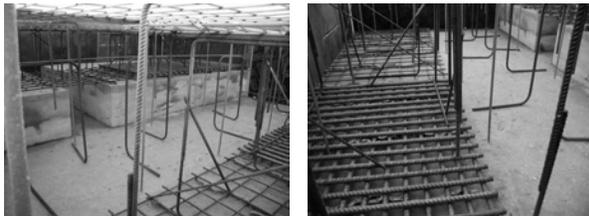
**Figure 3.** (a) and (b): Lean concrete layer and different levels of reinforcement before concreting (cf. (Taffe, 2008))
